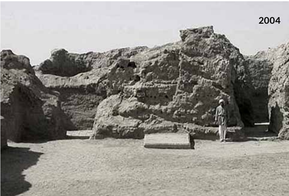
Examples of different types of events and processes that cause damage and loss of value to heritage assets. Weathering and erosion of earthen architecture structures at a heritage site over a period of 65 years (Royal Palace of Mari, Syria, between 1939 and 2004. Image courtesy of the Syrian Directorate-General for Antiquities and Museums).
