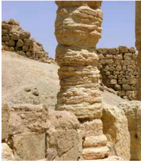
Wind erosion of a stone column in a heritage site (Image courtesy of Anwar Sabik, ICCROM).
