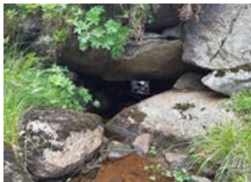
Examples of functional culverts made of stone. (Photo: Siv Annie Henriksen (left) and Håkon Aurlien)
