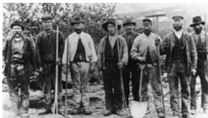
There are no photos from the construction of the road over the mountain. Here is a roadworks team at work on a cross-border national road further south in Nordland, around 1900.
