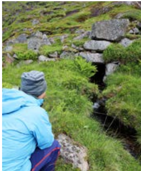
Examples of functional culverts made of stone. (Photo: Siv Annie Henriksen (left) and Håkon Aurlien)
