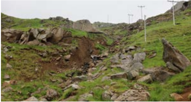
Here, parts of the old road have disappeared into a gorge formed by rockslides and water erosion. One of the rocks is lying at the very edge. (Photo: Håkon Aurlien)
