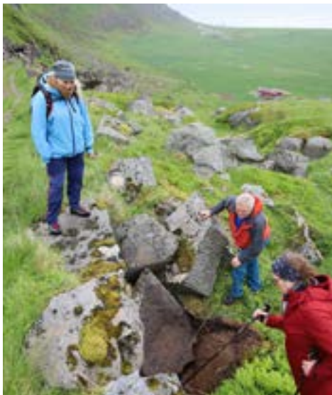
A partly collapsed culvert in need of repair. (Photo: Håkon Aurlien)
