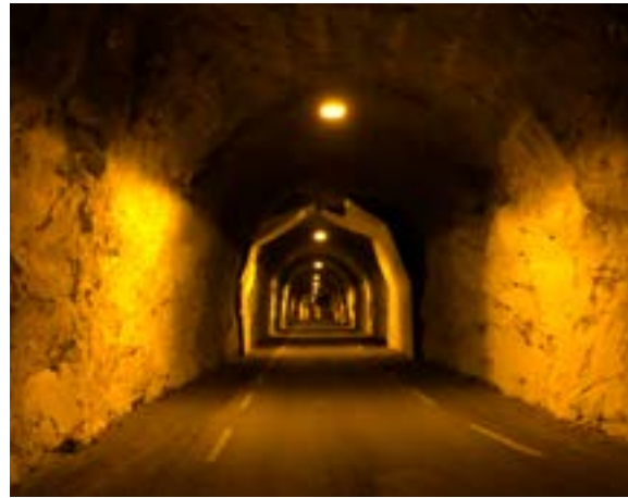
The Uttakleiv tunnel takes the local residents, and with time quite a few tourists, from Haukland Beach to Uttakleiv. The names of the 13 children who got a safer road to school are carved on a memorial plate dated 2 October 1998. (Photo: Håkon Aurlien)
