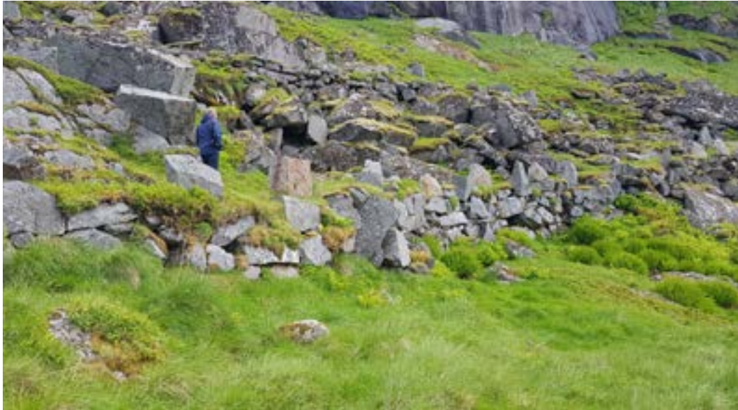
The road is built up in the terrain with dry walls, and lined with guard stones. (Photo: Ann Kristin Engh)
